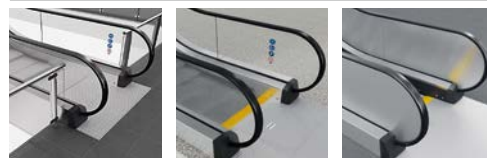
Extension de balustrade
